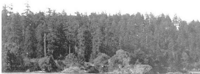
Figure 7: Nymph Point circa 1920 on the right opposite Mill Point to the left; the North Saanich dock is in the centre. Figure 8: Looking directly across from Mill Point to Nymph Point. Date is unknown but likely about 1930.
